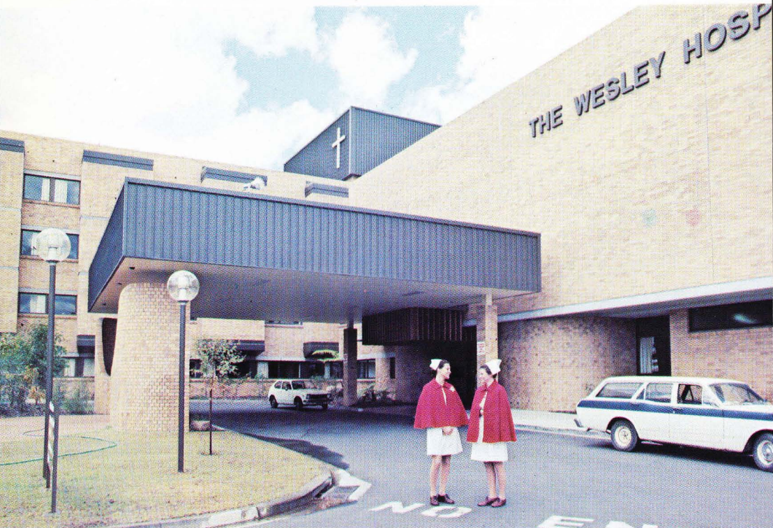
HEALTH—Chapter 8 Recently completed private hospital, Brisbane
